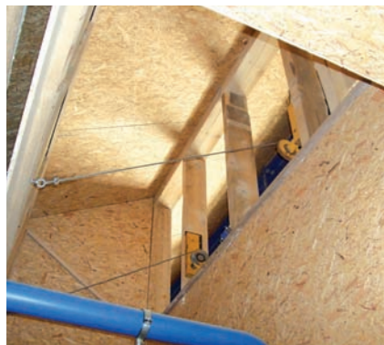
16 Recirculating air flap
